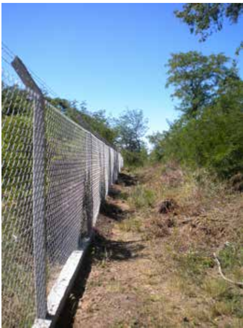
New perimeter fence
