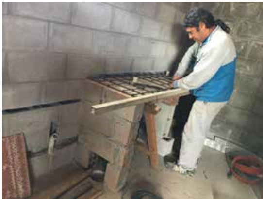
Construction of counter for sinks
