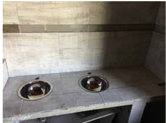
Bathrooms sinks near completion
