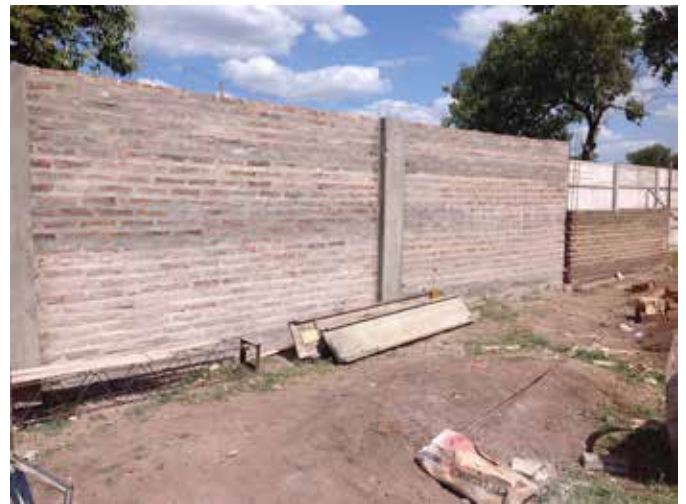
New brick wall
