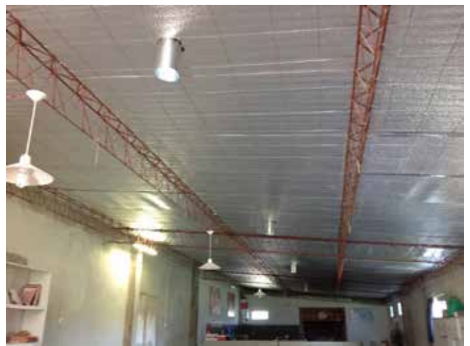
Kitchen insulation and ventilation
