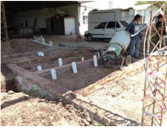
Foundations for bathrooms
