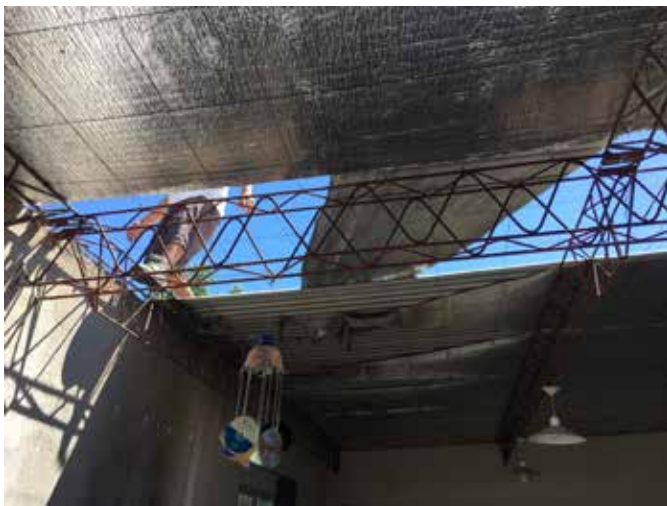
Kitchen insulation and ventilation
